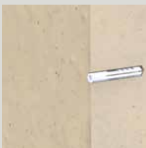
1. Insert suitable dowel into wall
